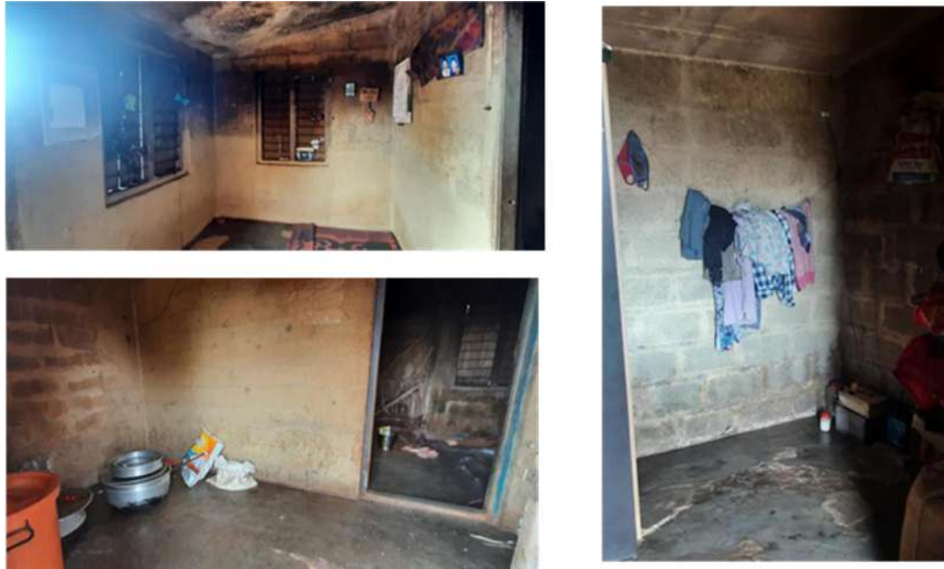
Figure 13: Typology 1 -Hollow Concrete modern Salai structure
