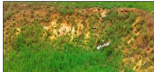
Site 2- Kankol Substation
